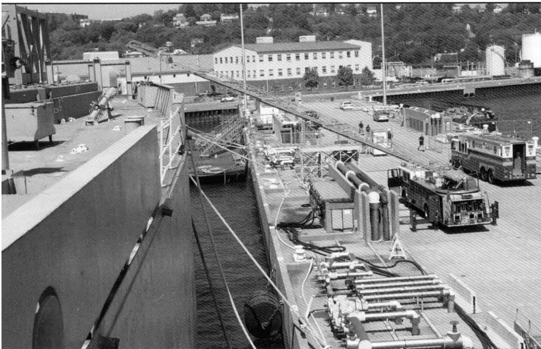
Training evolutions took place on the 950-foot-long Denebola . FDNY members developed an appreciation for the hazards encountered with shipboard fires.
